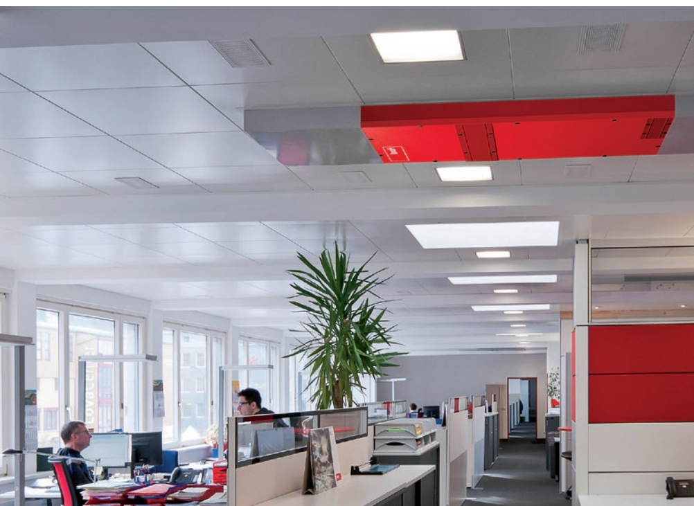
Visible technology in a suspended ceiling: As a decentralised comfort ventilation system, the Hoval HomeVent® is also suitable for renovations.
