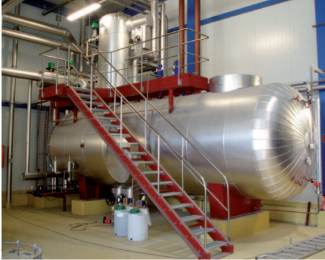
Feedwater tank with thermal deaerator
