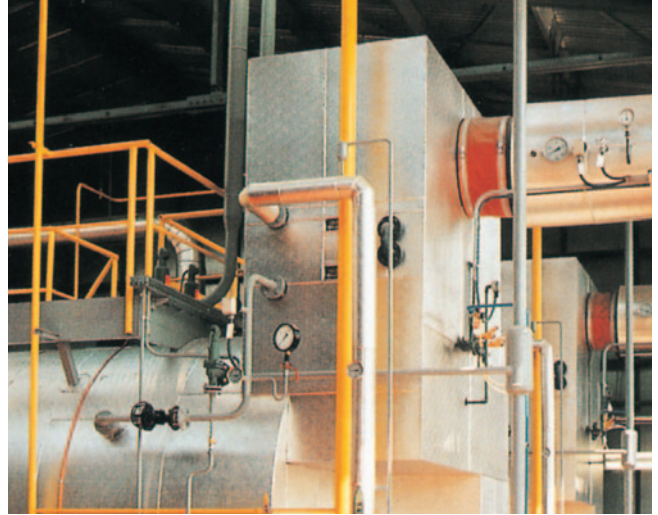
Flue gas heat exchanger and components for optimisation of efficiency
